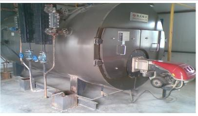
Boiling cleaning device: Heavy oil cleaning, steam boiler circulating heating 80-110 C, 150-180 pcs/4h per pool
